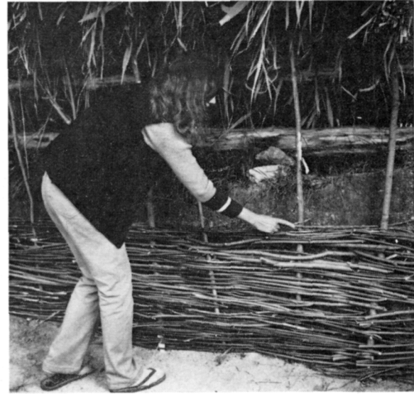
Fig. 7. House No. 5. Covering of the roof. 1 — thrusting a reed thatch onto a wooden sword; 2 — binding of thatch to horizontal sticks; 3 — S side of roof with wattle. Building of walls. 4 — wattling.
