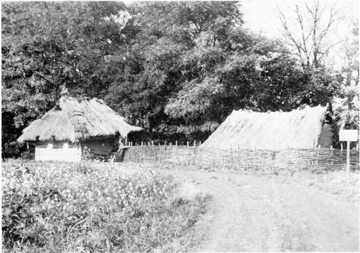
Fig. 41. Březno, district of Louny. General view of both experimental buildings.
