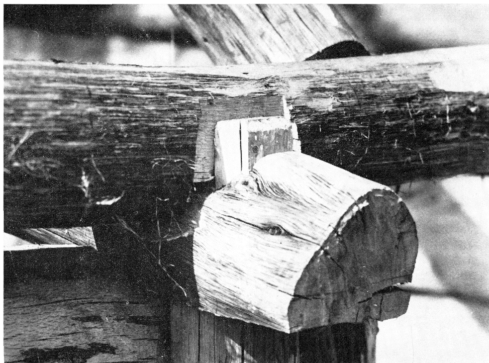
Fig. 19. House No. 69. Transversal trunk tenoned into posts at the entrance and rabbeted by the circle of round timbers.
