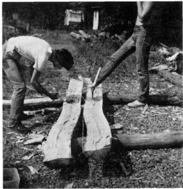
Fig. 13. House No. 69. 1 — 4 — cutting of trunks for building of the walls.
