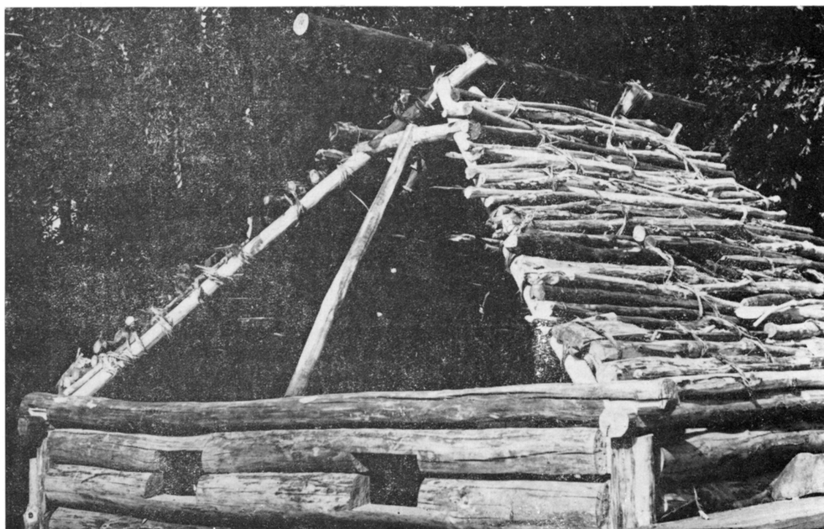
Fig. 21. House No. 69. 1 -- construction of roof (lower mantle); 2 -- lower mantle of the truss filled in by sticks.
