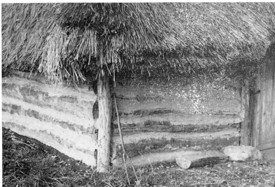
Fig. 26. House No. 69. 1 — interior of the structure — NW corner, gaps not yet filled in; 2 — SE corner with gaps filled in, outside view.
