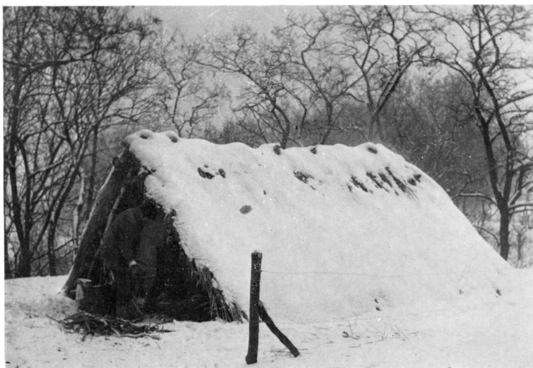
Fig. 31. House No. 5. 1 — evacuation of smoke through the ridge and upper parts of the roof; 2 — evacuation of smoke through the upper parts of the roof where the snow cover has melted in a strip.
