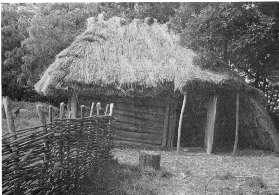
Fig. 25. House No. 69. 1 — covering of the roof by thatch of rye straw; 2 — view of the E side with the entrance.
