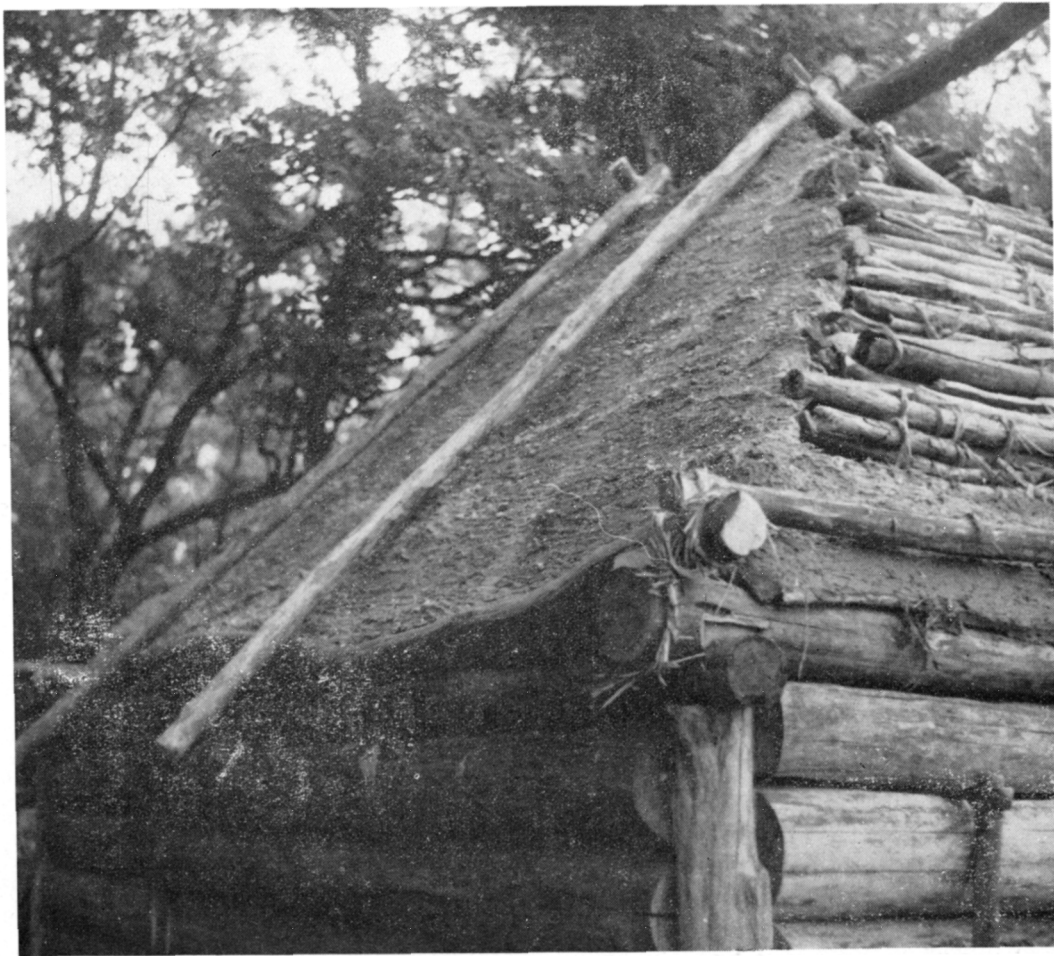
Fig. 22. House No. 69. 1 — cutting a shallow mortise into a rafter of the upper mantle of the roof by means of an adze; 2 — tying of rafters of the upper mantle by twines of willow twigs; 3 — clay daub on the sticks of the lower mantle of the roof.
