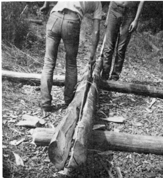
Fig. 13. House No. 69. 1 — 4 — cutting of trunks for building of the walls.
