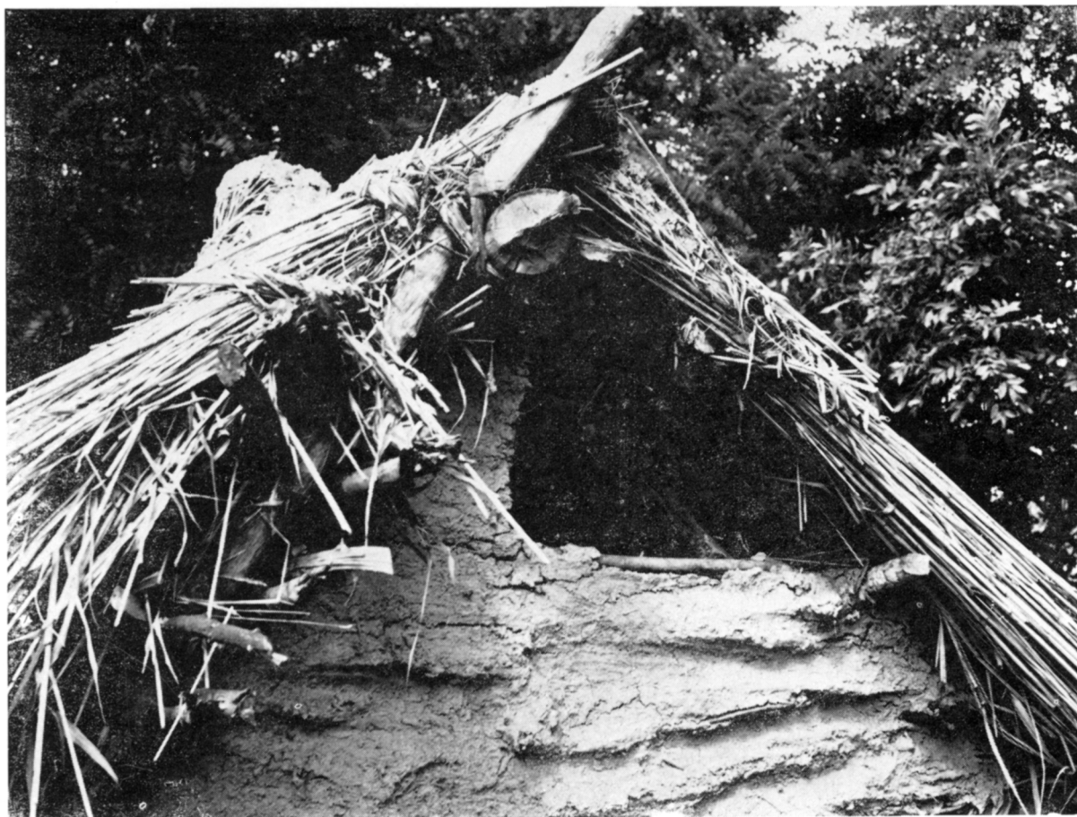
Fig. 8. House No. 5. Ventilation aperture in the E gable; daubing of walls.
