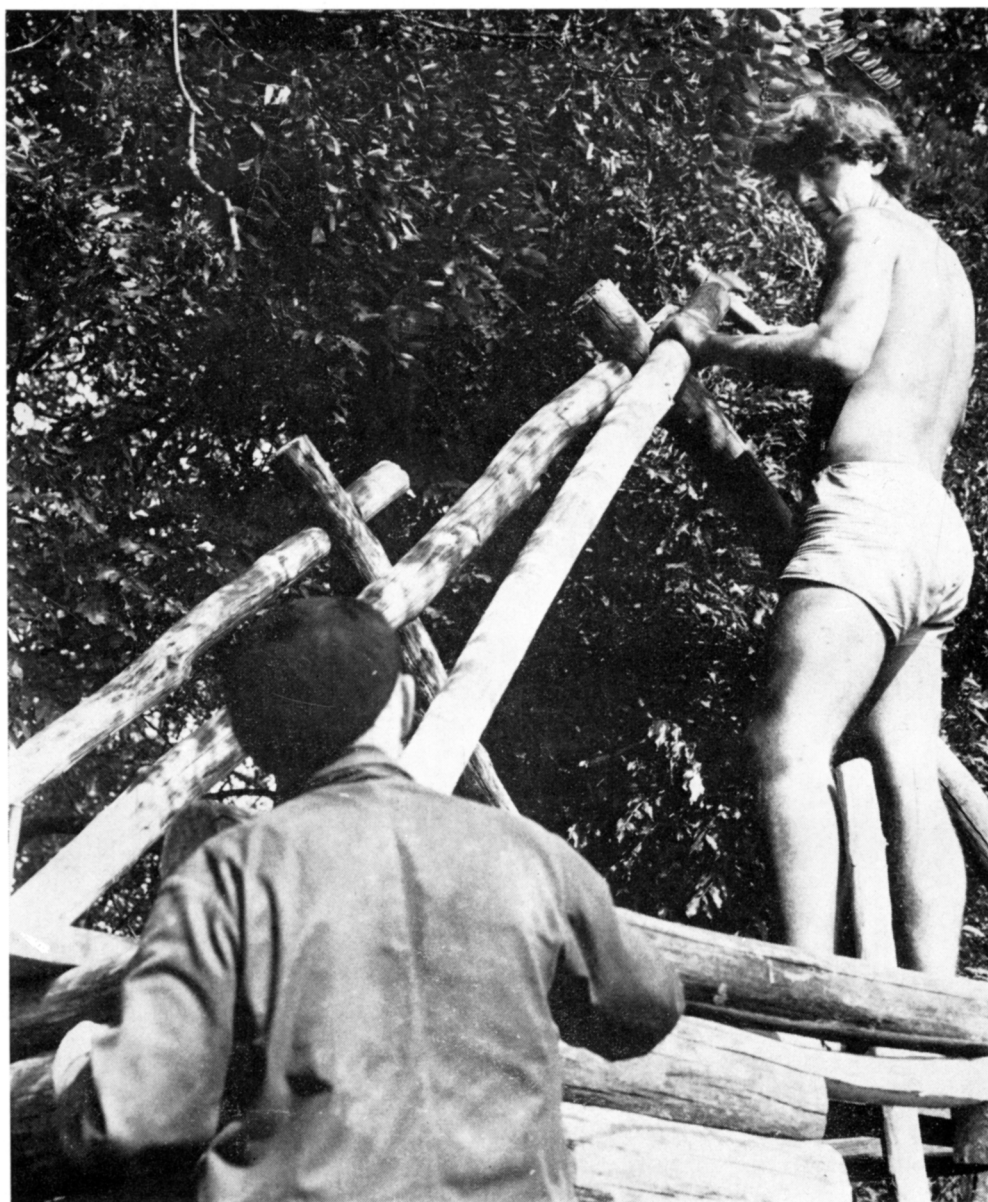
Fig. 20. House No. 69. Building of the roof.
